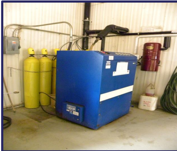
Air Compressor to Refill SCBA Bottles
