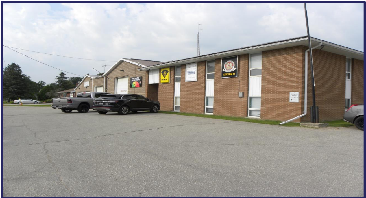
This portion was the original Township of Tosorontio Municipal Offices.
