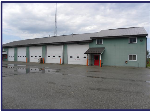
East side office area
