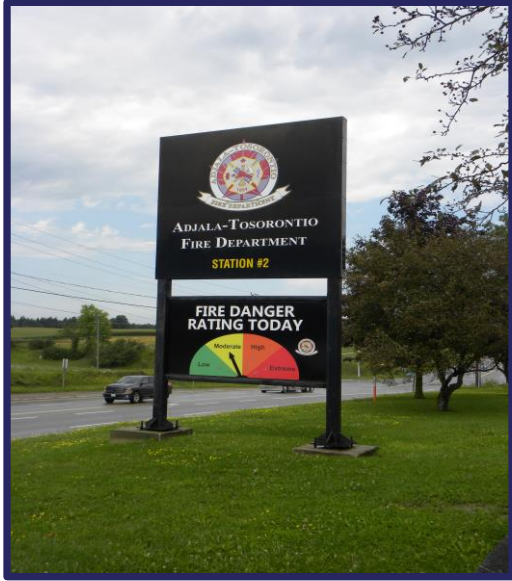
Front of Station 2
