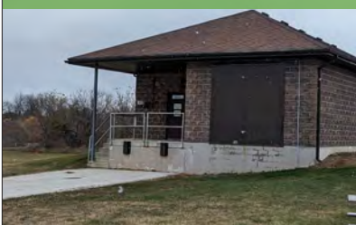
WATER TREATMENT PLANT
