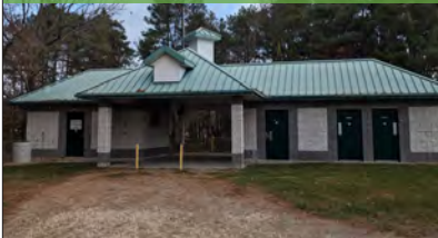
WASHROOM / PUMPING STATION
